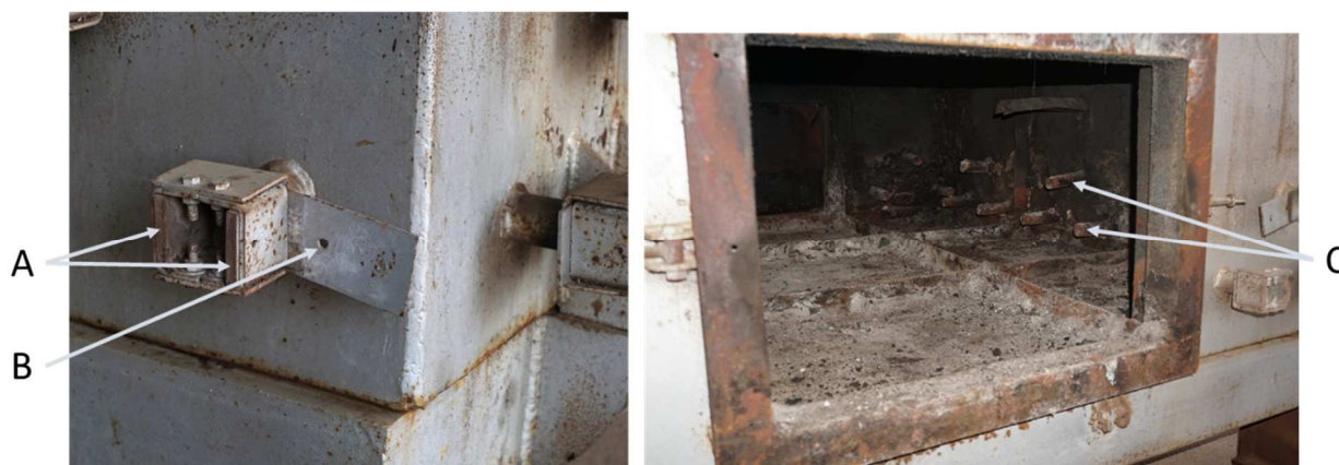
Figure 2 – External (left) and internal (right) views of the nozzle tubes with (A) permanent magnet positions, (B) drilled plate for the manual air flow adjustment, (C) nozzles tubes inside the combustion chamber.
